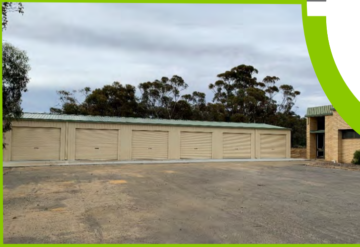
Newly installed 6 Bay Shed at Civic Centre
