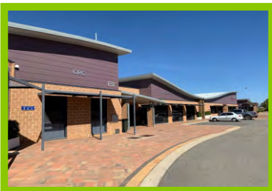
Before and after photographs: Community Resource Centre Exterior Painting
