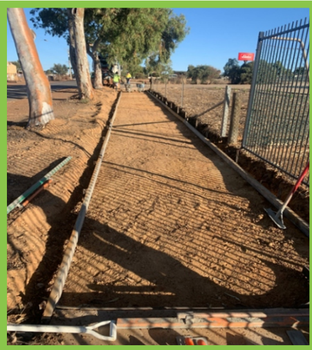
Footpath repairs Northam-Pithara Road
