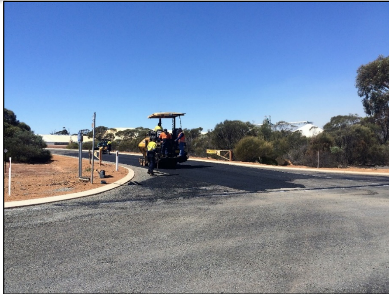
Intersection Repairs in Ballidu
