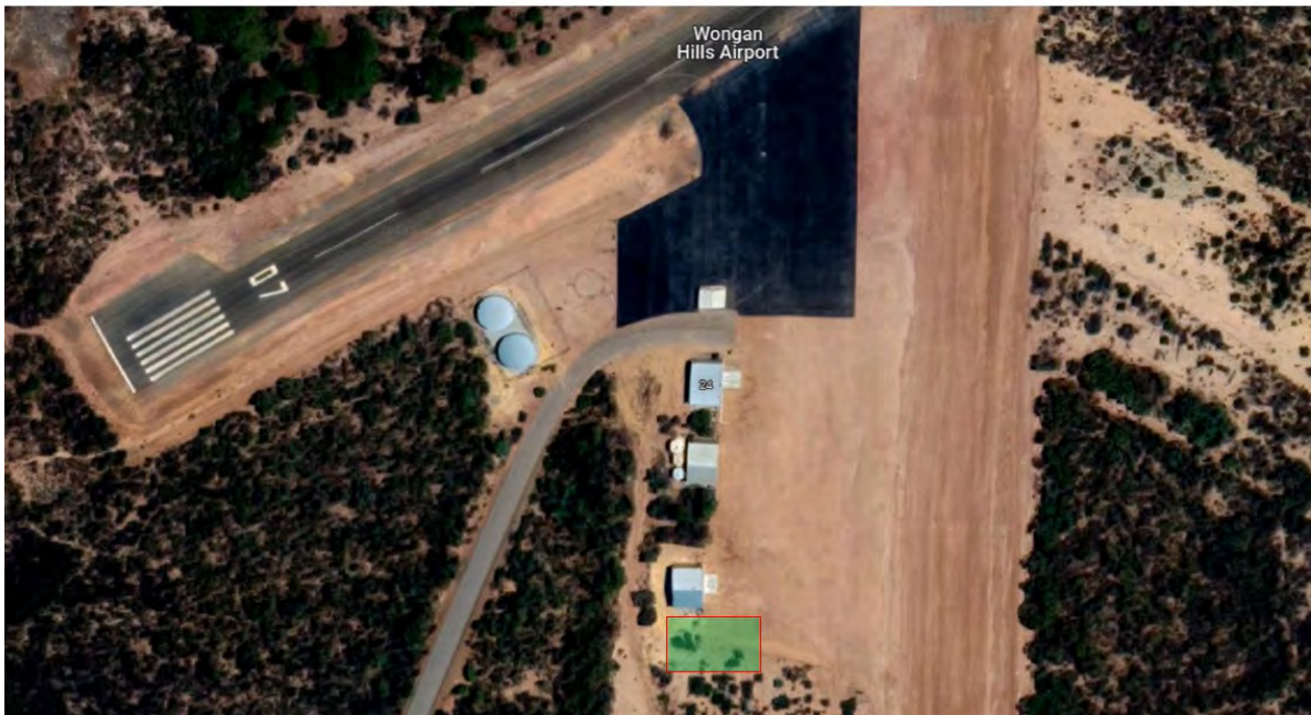
The site area to be cleared
