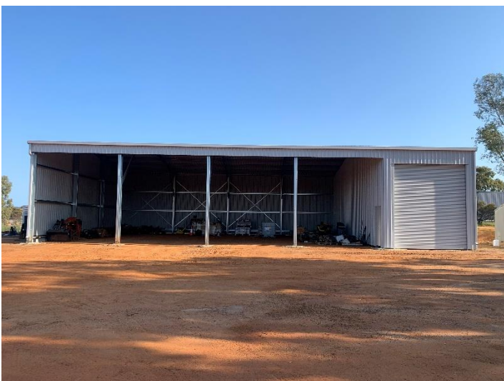
Shire Depot Machinery Shed
