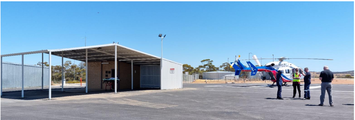
Wongan Hills Airport Shelter Upgrade
