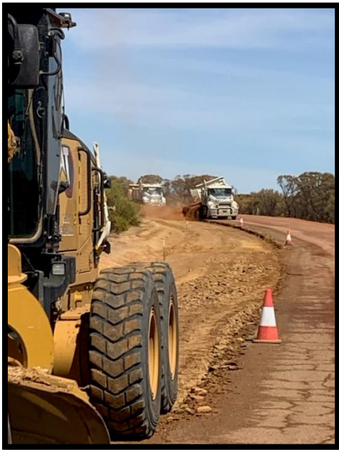
Road Widening Burakin-Wialki Road
