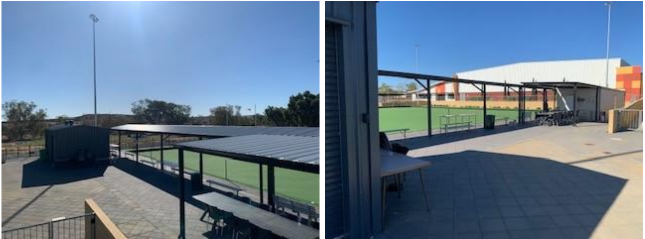
Photographs of site as at 20 March 2024
