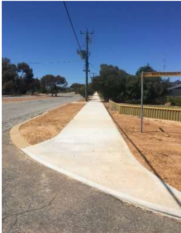
Footpath on Wandoo Crescent
